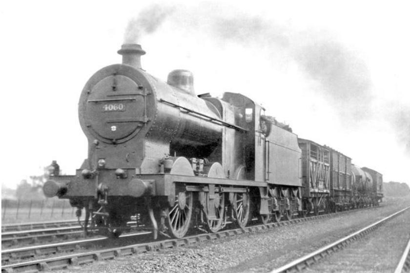
*A mixed milk train carrying churns and tank wagons c1932-34. 4F No.4060 is believed to be near Roade and behind the cattle truck (which could in an emergency be used to carry churns) is an ex-NSR milk van. Following are three tankers on 4w chassis built in 1931 for United Dairies, the first for 2000 gallons, the other two for 3000 gallons. On the rear is an ex-NSR 6w brake van. AUTHOR'S COLLECTION*
